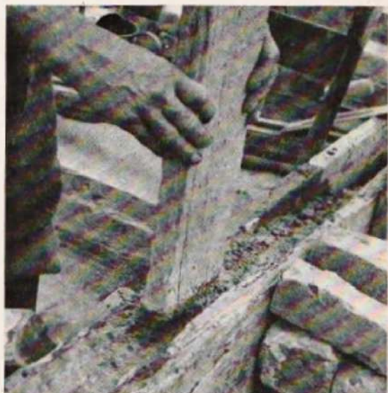
When the concrete is poured in between the shuttering it is pummelled so that no large cavities are left. If wood is used for shuttering it is best to grease or oil it very thinly initially.
