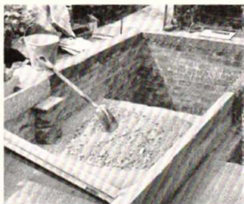
Above: The dry ingredients of the concrete are very thoroughly mixed.
