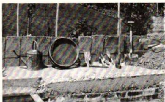
Above: Tools used for pond building. Behind them are breeze blocks which can be temporarily employed as shuttering material.
