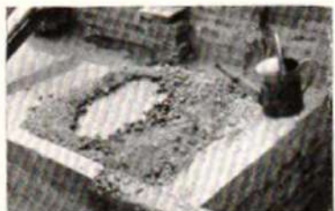
Above: The dry ingredients of the concrete are very thoroughly mixed.
