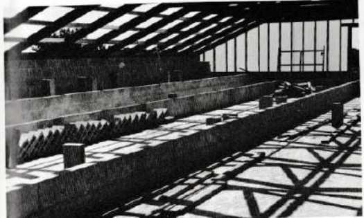
The inside of Gulf's new plant research building which will be under the supervision of Heiko Bleher. This building will feature huge concrete vats for cultivating new and rare aquarium plants as well as for growing many common varieties. The pools are made of 4"-concrete blocks which are slotted with cement to bond them together. The pools are of various heights to control the growth of the plants more uniformly.
