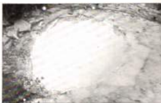
...nearly ready for the liner.
