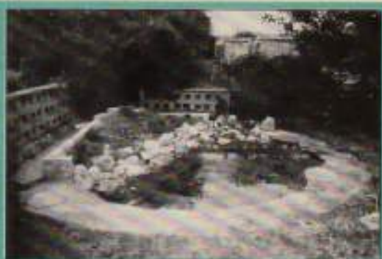
The completed pond.
