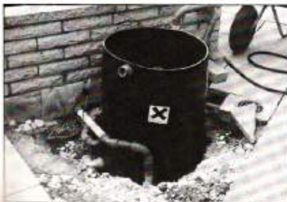
The settlement chamber before bricking in.
