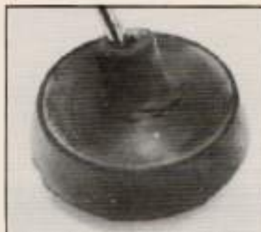
The diaphragm may seem OK at first sight but if you twist the fixing shank the split will be obvious.
