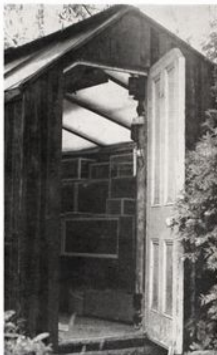
A garden fish house entrance showing features mentioned in the article (multiple glazing, draught strip etc.). Check meters are seen to the right of the doorway
