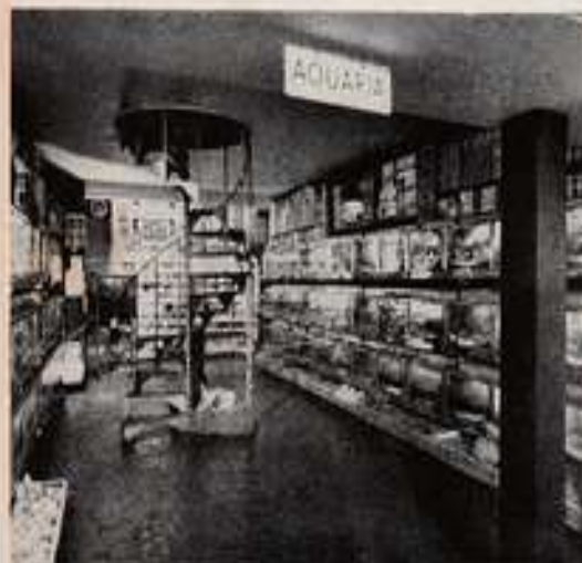
View of the ground floor Aquaria Section with all stainless steel tanks
