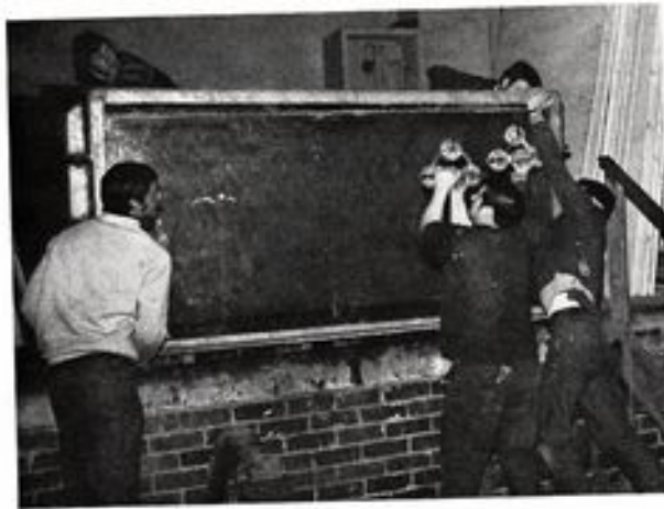
Glaziers fit a 6 cwt. glass panel into one of Liverpool Museum's new fibreglass tanks, helped by Keeper Denis Murphy (left)
