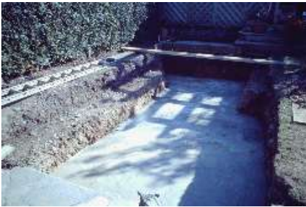
3. Give plenty of time for concrete to set
