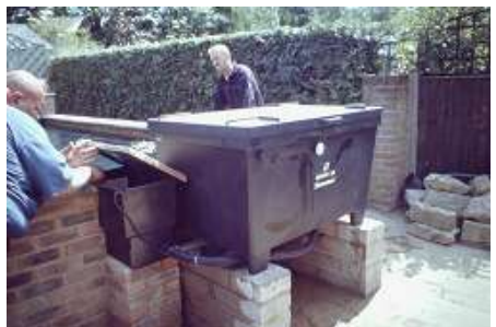
12. Pumps in place and working.
