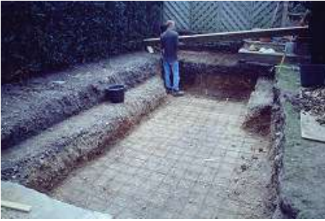
1. Excavations complete with wire reinforcements
