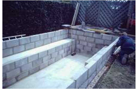
8. Bricklaying the outer wall (note wire ties)
