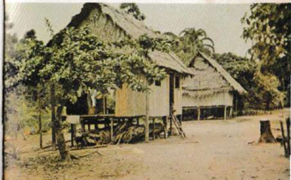
The houses of the Ticunas are up on stilts to keep them dry when the Amazon overflows its banks.
