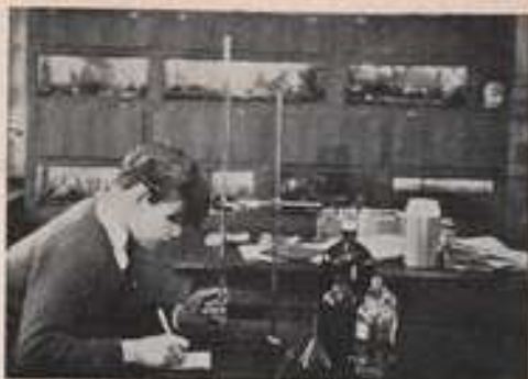
Water testing is done regularly. Here a pupil is seen estimating water reaction by a bromothymol blue test.
