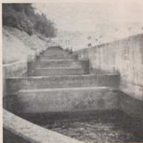
Photograph 1: a fish ladder
