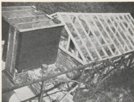
The fish house complete
