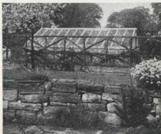
The author's completed fish house, seen beyond a dry wall and trellis
