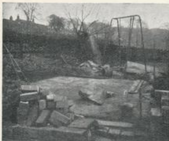
Materials begin to arrive at the site, which is being cleared
