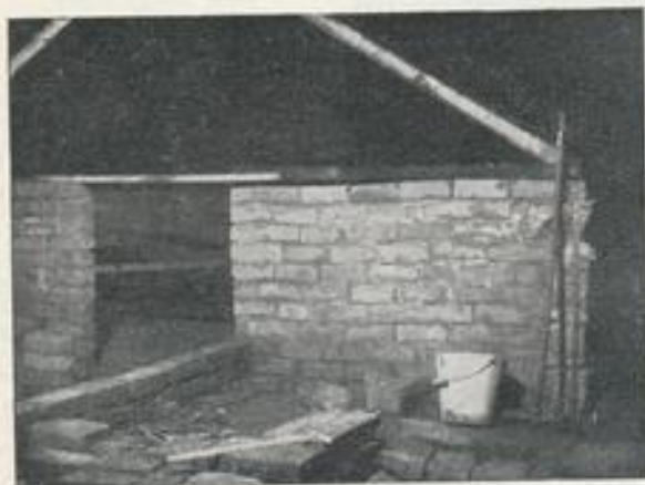
First stages in the timber construction of the fish house
