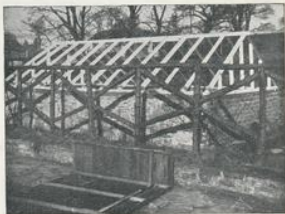
Completed roof timbering of the fish house seen from the side
