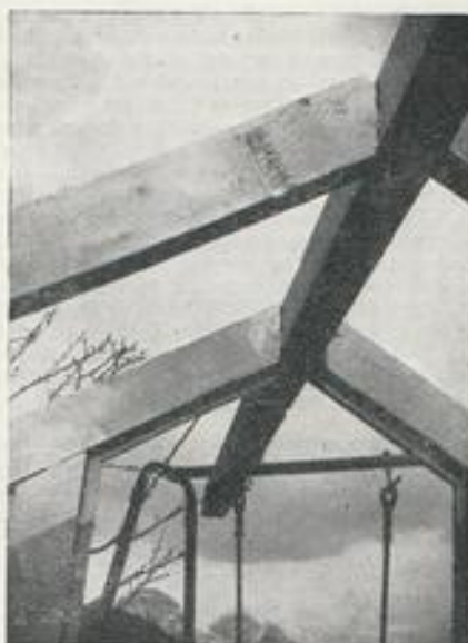
View of roof joints from within the fish house
