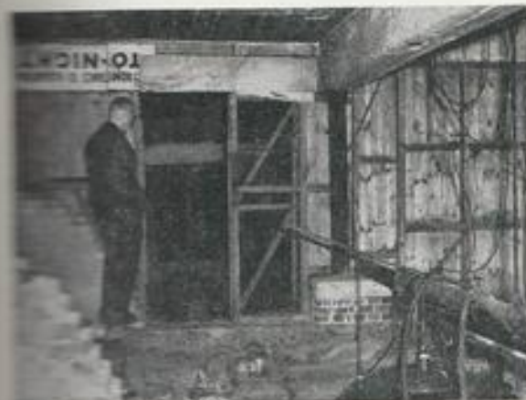
View the tanks—once a platform of planks spanned these for efficient servicing, but this has long since disappeared and has never been replaced
