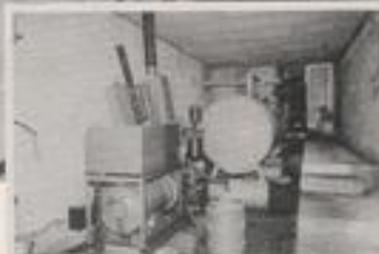
Behind the scenes, Mallorca Aquarium, where pressure filters clean the water in the Show Aquaria
