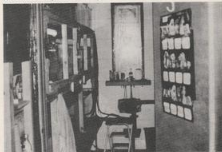
Photograph 2 shows the interior of the fish room as photographed from the work area. Note the small window installed in the end wall and the inevitable condensation despite the double glazing
