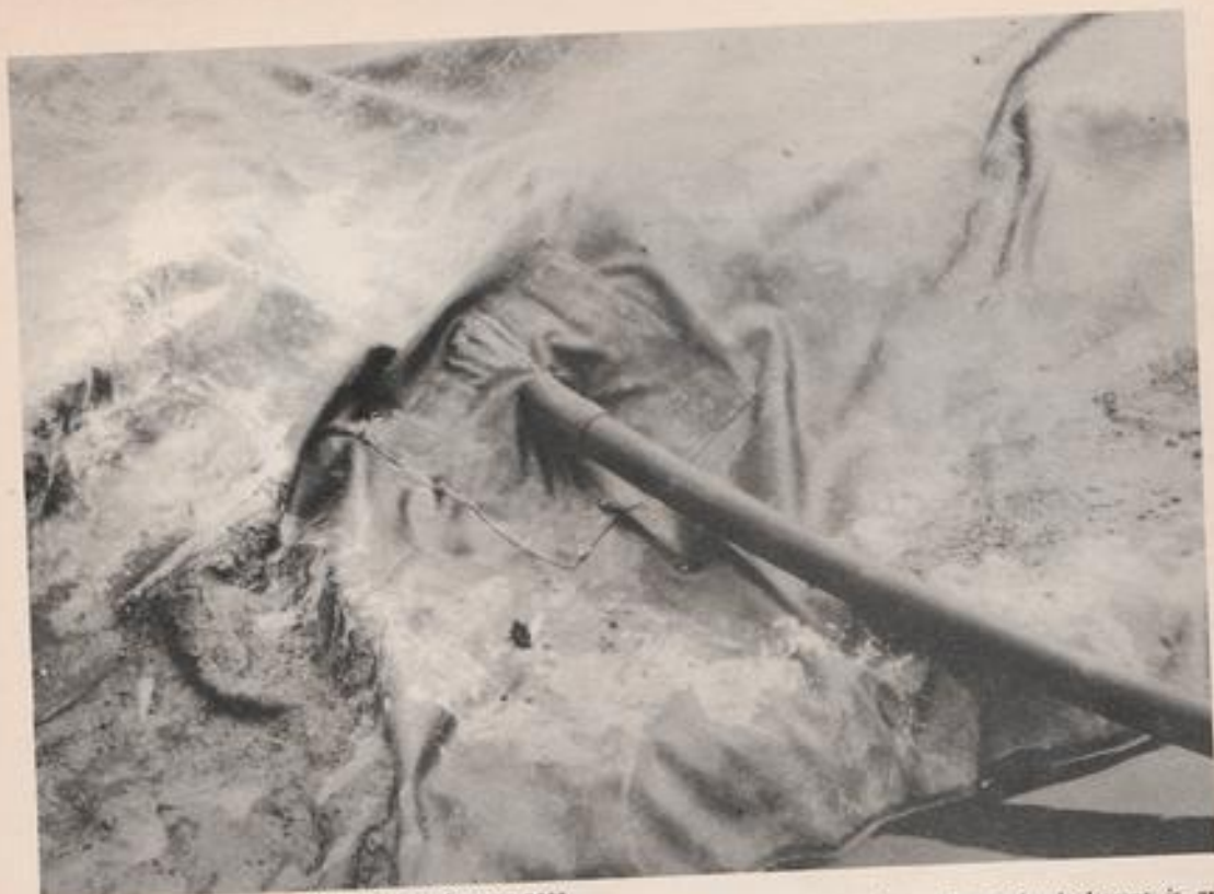
Close-up of flange (sleeve) by which a pipe can pass through Butyl Rubber
