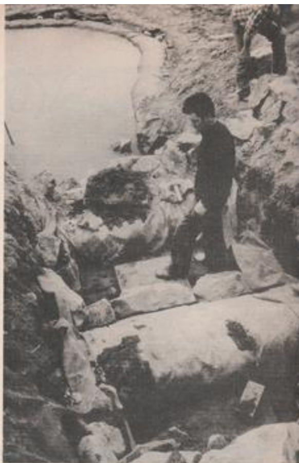
Waterfall during construction
