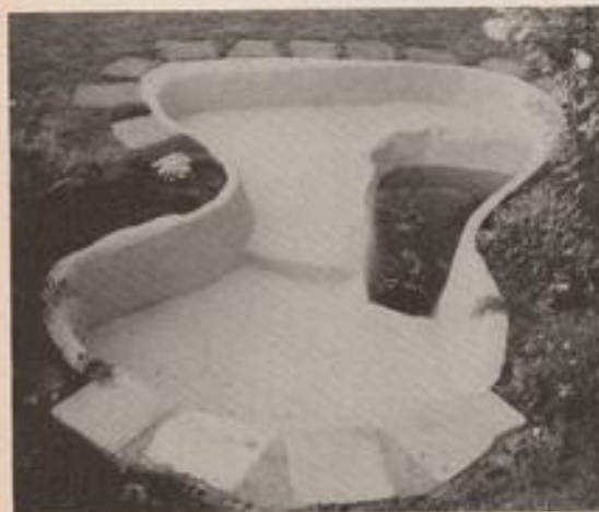
Informal concrete pond with three different depths.
