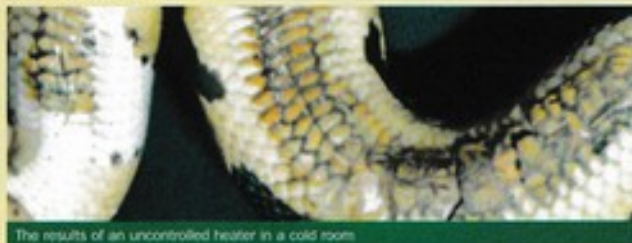
The results of an uncontrolled heater in a cold room
