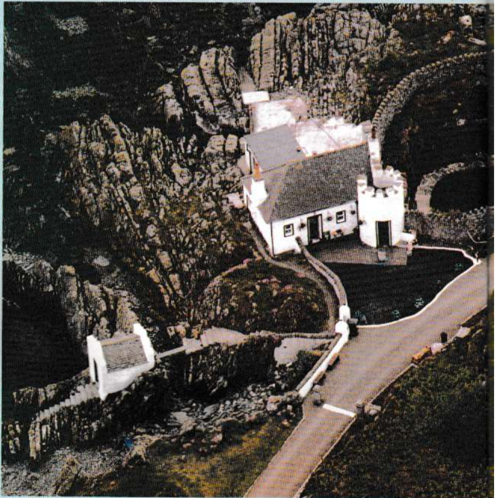
► An aerial view of the Logan Fish Pond Marine Life Centre.
