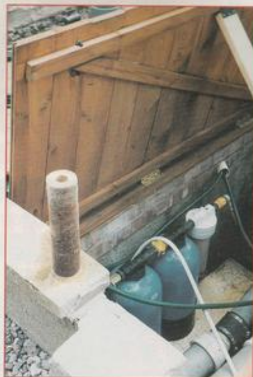
ABOVE A three stage water purifier with used sediment filter on display.
