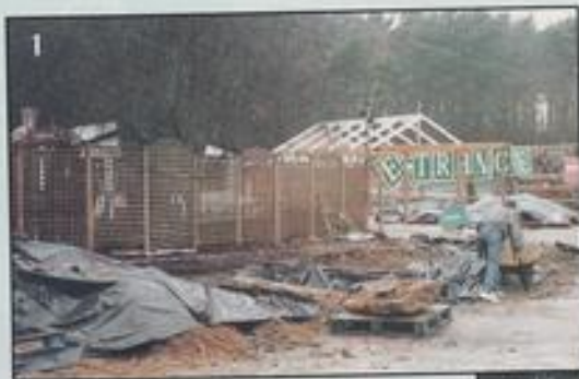
1 The physically hardest work is digging the hole.
