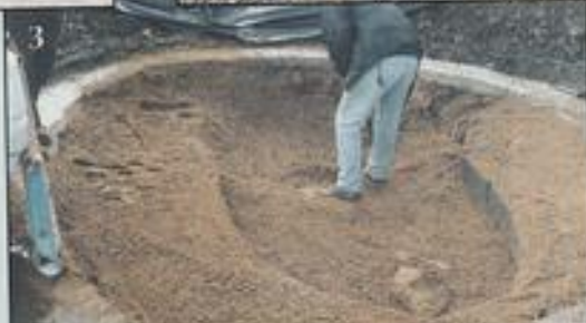
4 Linderlay is also used on difficult to cover areas before laying down the liner.
