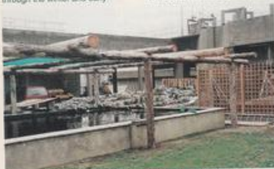
The pond nearing completion under the shadow of the treatment works.
