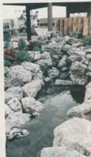
The water course almost ready for planting.
