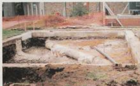
The massive 18-inch steel air pipe.
