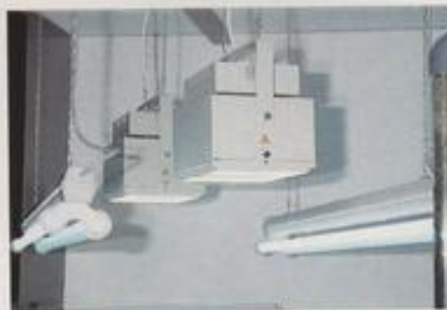
A look behind the scenes of the German office aquarium. Metal halide lamps and actinic blue fluorescent tubes have been used to create the appropriate lighting.
