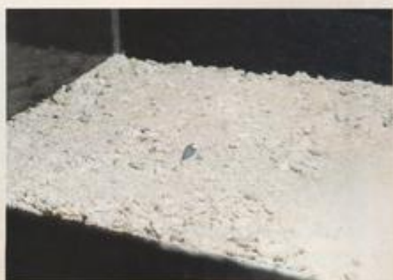
Filter matting is laid over the egg crate, followed by a layer of clean 'virgin' sand.
