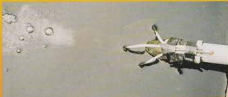
A Venturi return of water to the pond provides an effective means of aerating the water. These devices are particularly useful during high summer.
