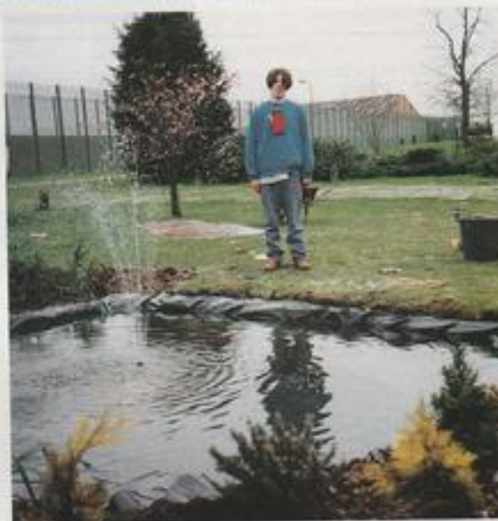
TOP — The pond project nears completion.
