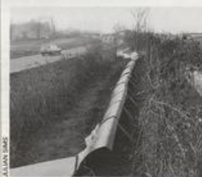
The ACO Amphibian Fence. Shelter is provided by this concave barrier which is supported by plastic poles. In the foreground is a conventional drift fence made from polythene sheeting.
