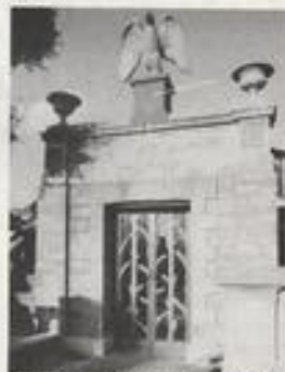
Entrance to Bristol Zoo's World of Water which is 'plumbed in' using Durapipe ABS.
