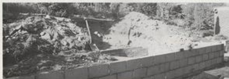
Pond Building need not be difficult. Here, a sloping garden (mine!) is walled and concrete-lined to create two ponds.
