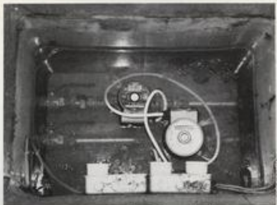
The price of complacency — a flooded pump chamber.
