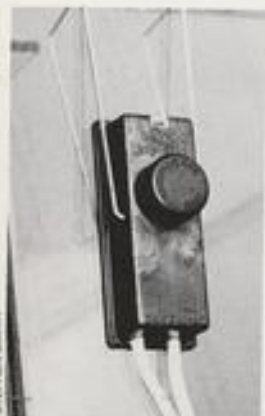
External thermostats usually clip on to the outside of the tank.
