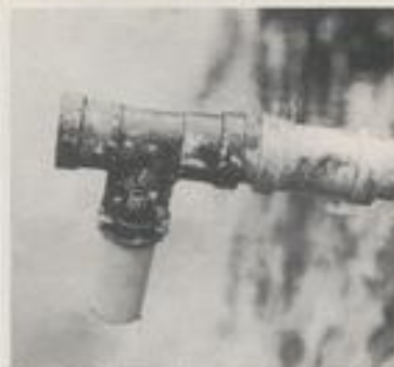
Above left. Venturi in summer mode — air is drawn down and pumped into the pool.
