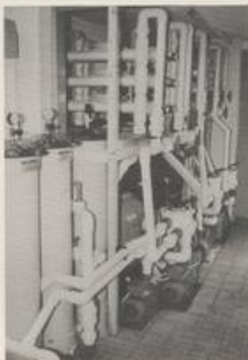
Part of the highly efficient filtration system at the Tropical Marine Centre
