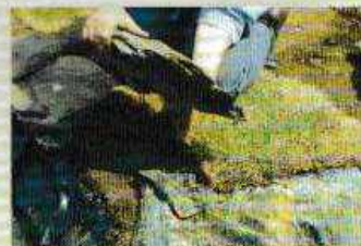
Step 5. Trim around the liner to make the edge neat and add slabs or turf to join the bog garden to the pond
