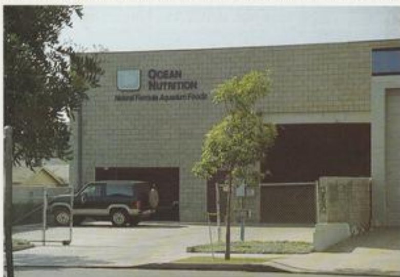
Ocean Nutrition's office and manufacturing unit photographed from the forecourt of the shipping and receiving warehouse.
