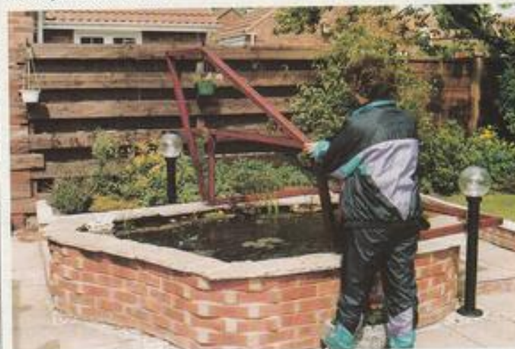
As a first step in removing the cover, the left hinged 'flap' is lifted.
