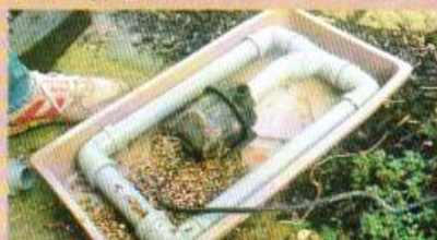
3. A tray goes under and around the unit.
