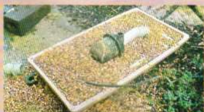
4. Topped-off with gravel the pre filter should not need cleaning more than once a year.
