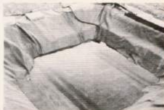
The Butyl sheet pool being filled.
