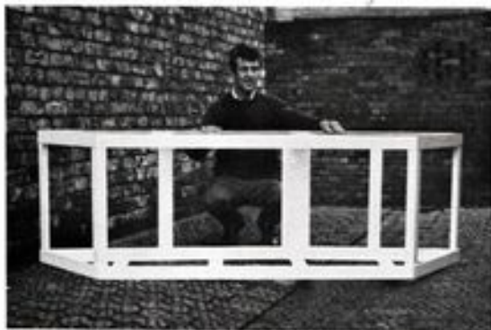
Frame of the aquarium before glazing. In this Monaco-type aquarium because of the angled ends it is not possible to see the tank corners from the front (nearest camera) when it holds water
