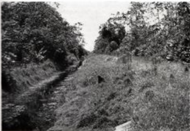
Drainage channel in the vicinity of a sugar cane plantation in Guyana, which was overgrown with Lophocorpus and Cabomba
