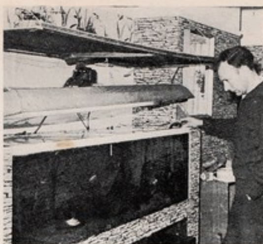
Mr Bell's lounge aquarium (six feet by 18 inches by 18 inches) with the cover closed (left) and raised (right) to show the overhead fluorescent lighting and also piston pump aerator
