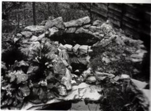
Brian Furner's waterfall and rockery pool photographed immediately after its construction with pieces of plastic liner sheet left over from the main pool. Rock plants will eventually mask gaps and edges in the surround.
