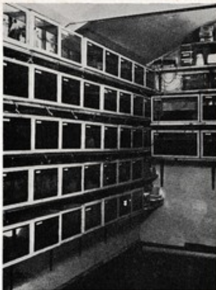
Small lightweight aquaria can be staged close together on metal brackets screwed to supports attached to fish house wall
