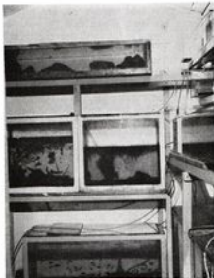
View within fish house to show wooden staging (right and top) used as well as an angle-iron stand
