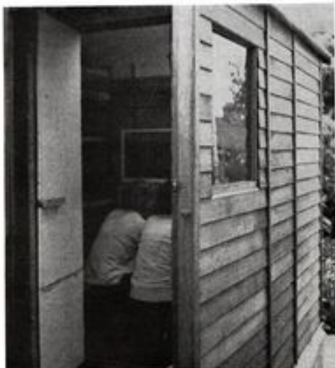
The doorway leads to a small garden store/heat trap section into which the white door of the tank section opens
