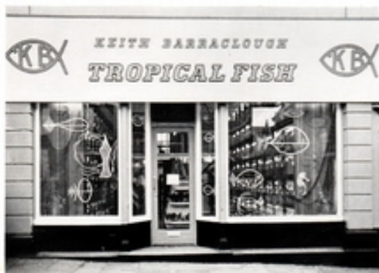
New Premises from Outside
