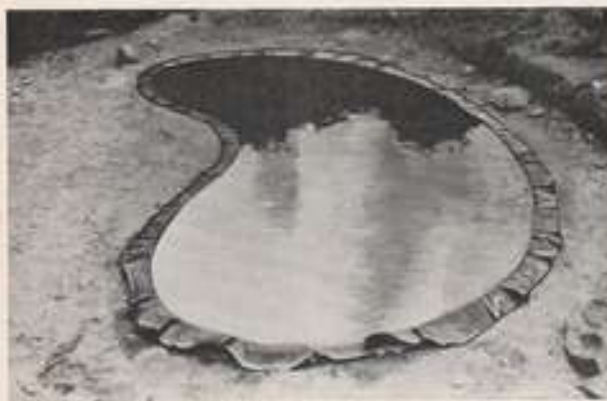
Butylite sheet is draped into the excavation and weighted at the edges. Weights are eased as the pool is filled so that the liner fits snugly. After filling (below) surplus sheet is trimmed to leave a 3-4 in. flap.
