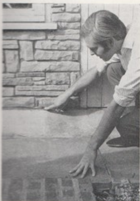
A damp-proof layer is placed on a thin layer of mortar immediately above the concrete raft of the fish house. Brick or stone courses are then laid
