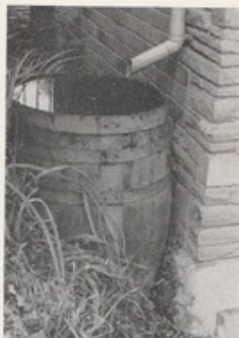
Collection of soft water—the easy way! Plastic pipes are used
