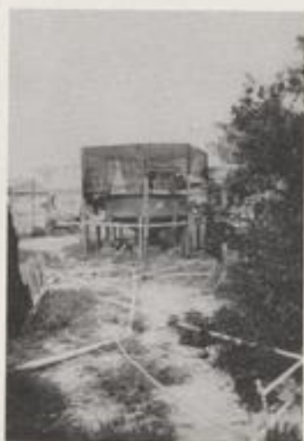
Raw sea water is taken from near shore and pumped to a huge sand filter in the first stage of preparation. The filter removes particles and parasites
