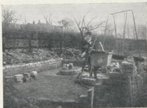
Concrete-mixing on the fish house site
