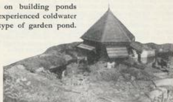
The turret-topped hexagonal observation chamber in the midst of Mr. Hounsfield's ponds
