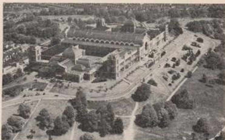
Alexandra Palace and Park. Photo: Aerofilms Ltd.
