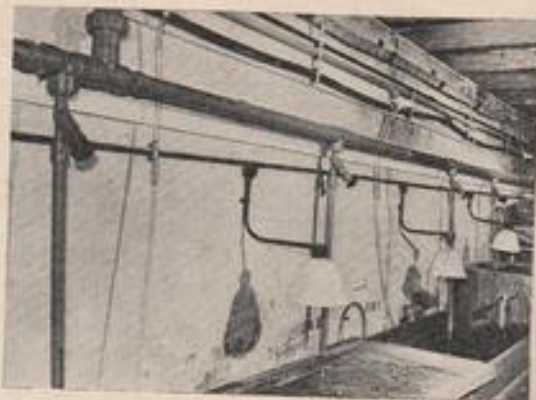
Fig. 2 The back of the amphibian tanks at London Zoo's aquarium. In this section, approximately 1,500 g.p.h. of fresh water flows through 500 ft. of Durapipe ABS.
