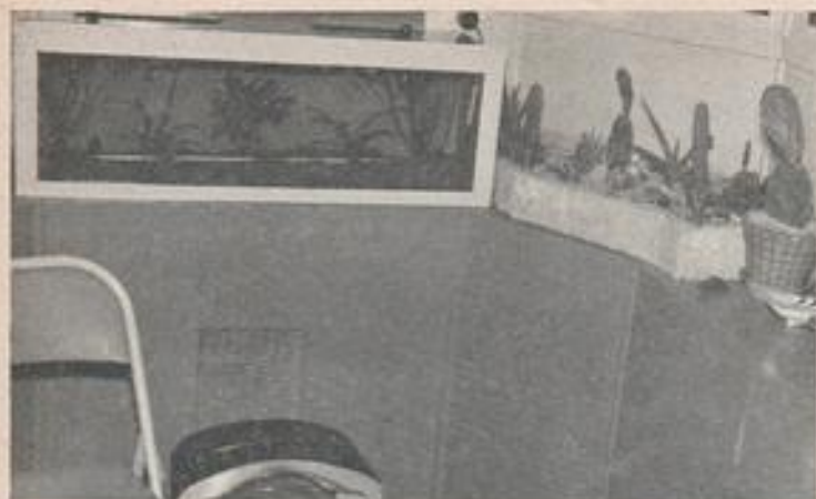
An opening of the fresh air duct that runs beneath the staging is seen beneath the large aquarium and in front of it is an oil heater for use on cold nights
